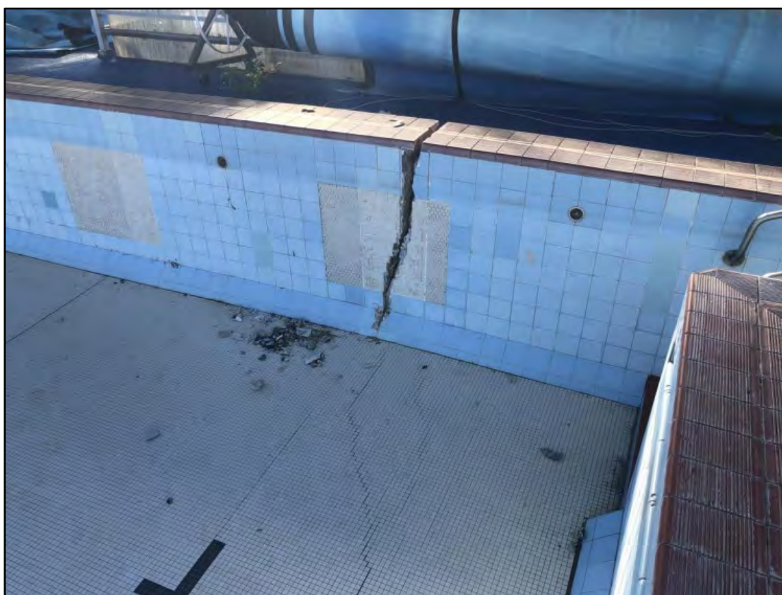
Figure 6 View of existing pool cracking at the northern end of the Olympic Pool
